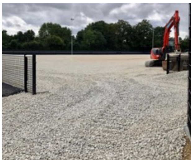
Hardcore laid over the pitch area, ready for a Tarmac covering and then 4m x 4m artificial turf sections
