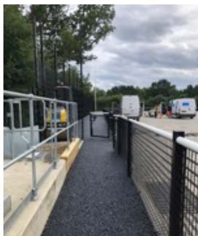
Spectator walkways laid with Tarmac over hardcore.
